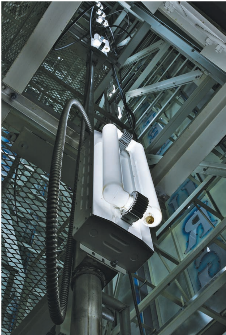
A peek inside the St. Petersburg sign structure shows how the lamps are placed inside.
